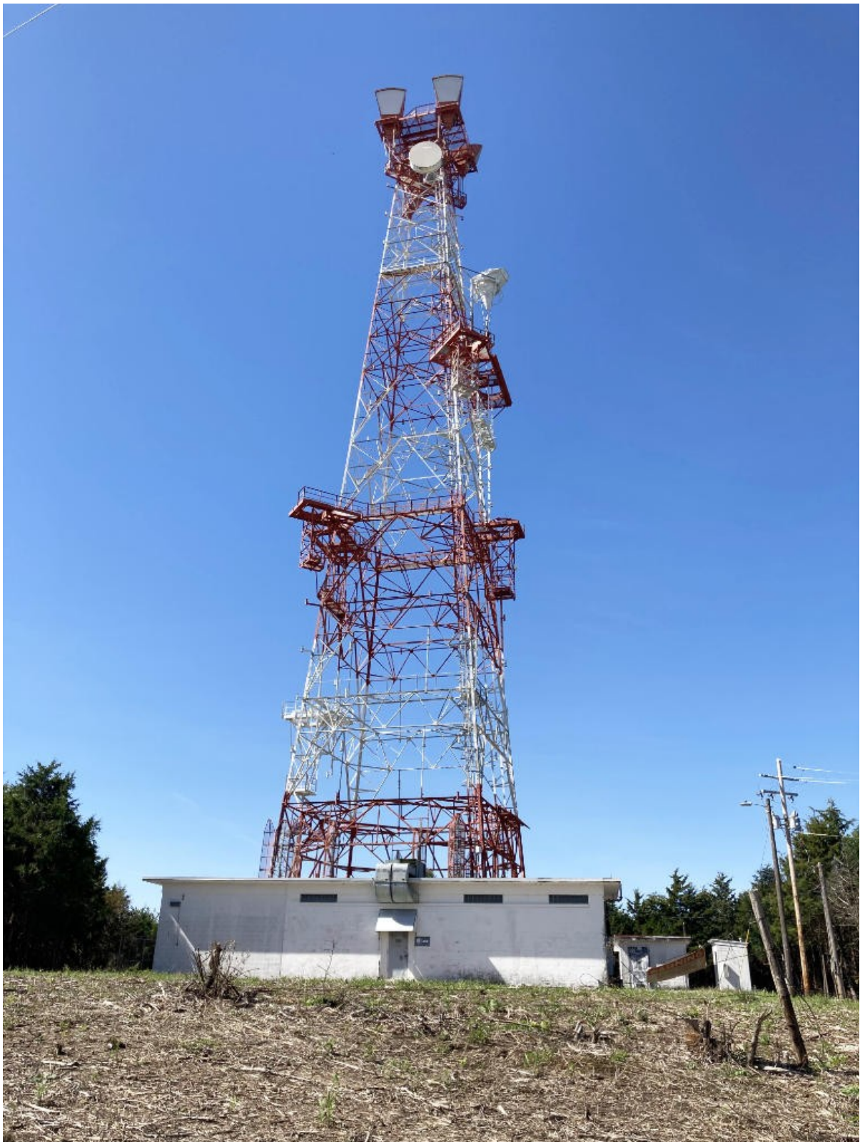
Site as viewed from Greenway Drive.
